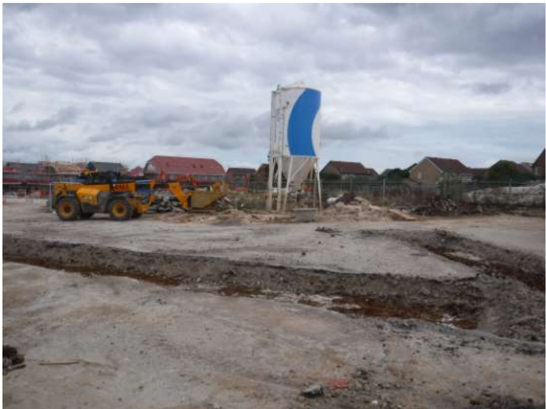
Plate 15 Concrete silo in use during evaluation.
