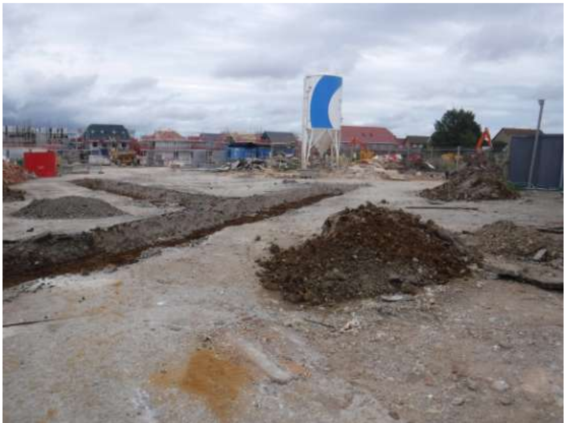
Plate 13 Overall view of site showing concrete silo at the center of the site.
